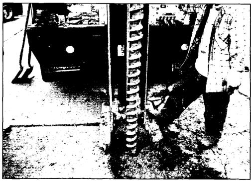
View of contaminated drill cuttings from MW-2.
